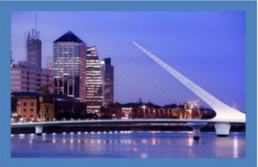
Buenos Aires Bridge
