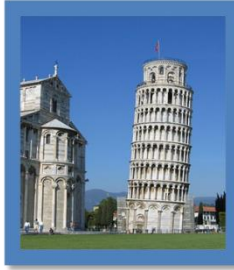
Leaning Tower of Pisa
