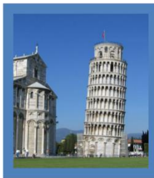
Leaning Tower of Pisa
