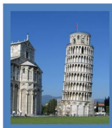
Leaning Tower of Pisa
