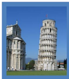
Leaning Tower of Pisa
