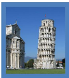
Leaning Tower of Pisa
