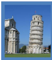
Leaning Tower of Pisa
