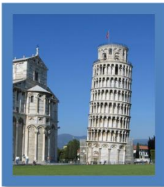
Leaning Tower of Pisa
