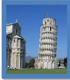
Leaning Tower of Pisa
