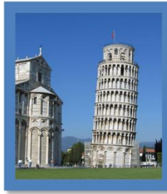
Leaning Tower of Pisa
